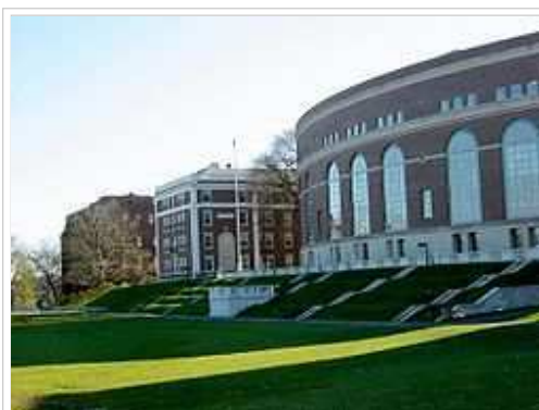
The view from Foss Hill. From left to right: Judd Hall, Harriman Hall (which houses the Public Affairs Center and the College of Social Studies), and Olin memorial library.
